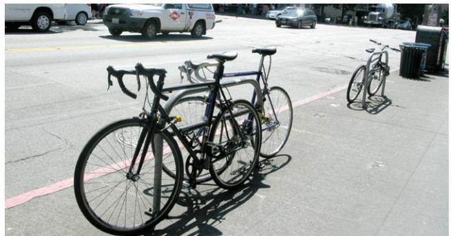
Rail type sidewalk racks on 1st Ave (Photo: SDOT)
